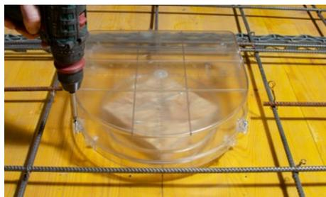
**3.** Attach the upper part of the back box using 4 screws.
