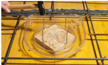
**2.** Position the lower part of the speaker back box and fix in place with 4 nails. (Take care when fixing in place and only hammer in nails until they are flush with the top of the back box.)
