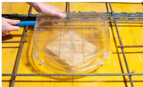
**4.** Connect the cable conduit. (Take care to avoid large gaps between back box and conduit)
