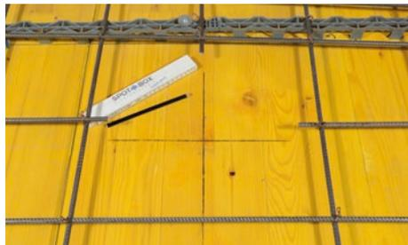
**1.** Determine desired location in the ceiling and mark position on cast.
