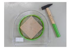
**2.** Position the lower part of the speaker back box and fix in place with 4 nails. (Take care when fixing in place and only hammer in nails until they are flush with the top of the back box.)
